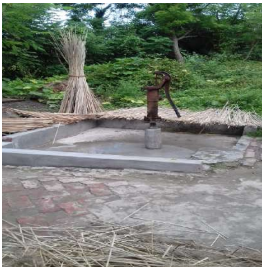
Damaged during Amphan
