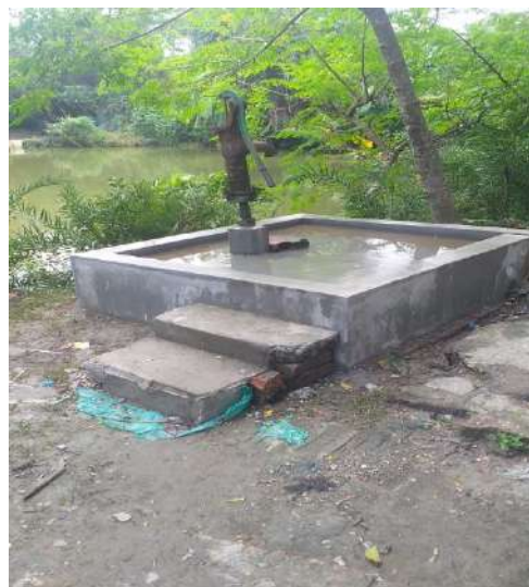
Repaired by SWS
